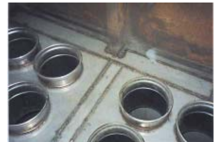
Installation of New Floors
