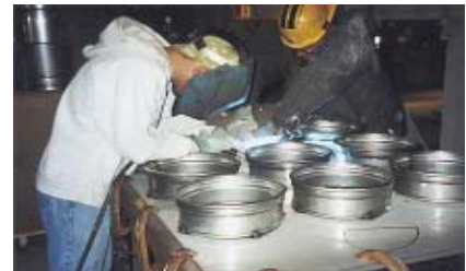
Fabrication of New Floors & Thimbles
