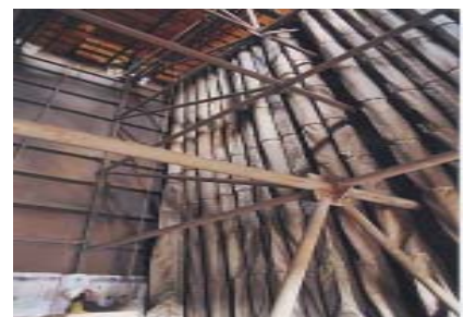
Installation of New Filter Bags
